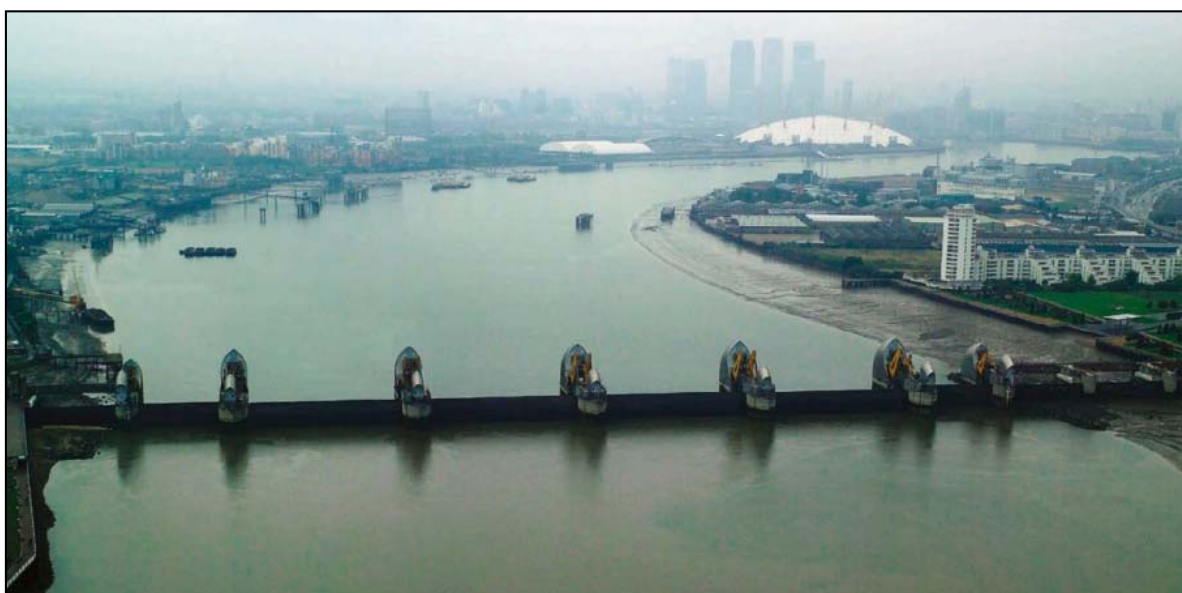
Figure 4.2 – Thames Barrier was built in 1982 in the Woolwich area to protect London from tidal surges (Source: Environment Agency, 2012a)
