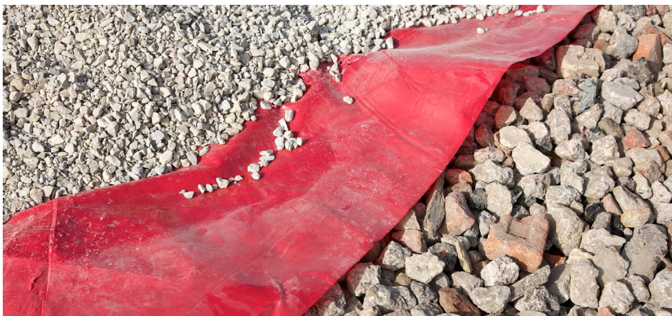
Figure 3. Example of lined permeable paving system. © Marshalls
