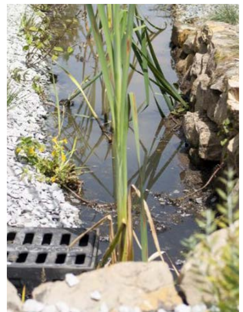
Figure 4. Recently installed Hydroplanter Flex System and Green Blue Urban Head Office. © Blue Green Urban
