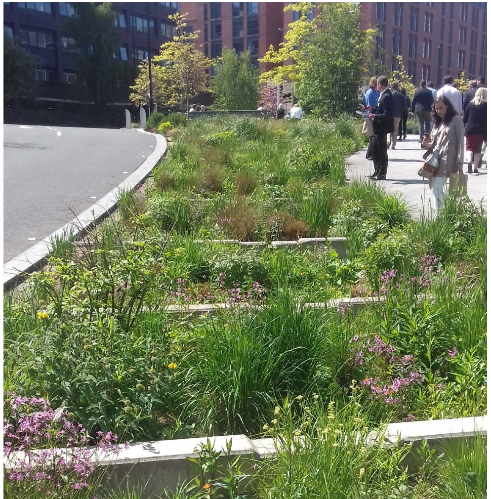
Figure 2. Sheffield Grey to Green Project showing concrete check dams. © Faye Gennard
