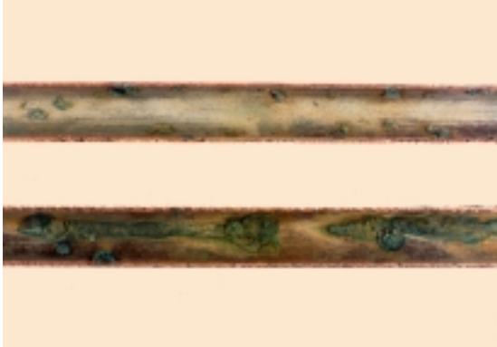
Photograph 1. Typical distribution of Type I pits in copper pipe
