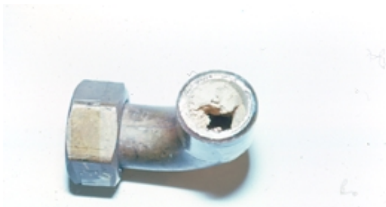
Photograph 5. A Brass fitting partially blocked by meringue dezincification
