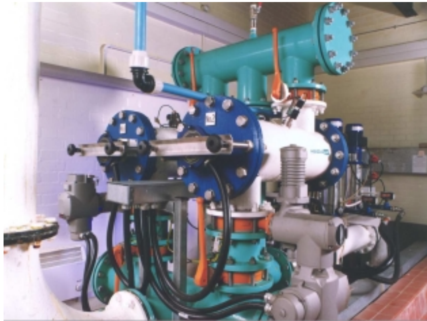
UV disinfection equipment. Photograph courtesy of Hanovia Ltd.
