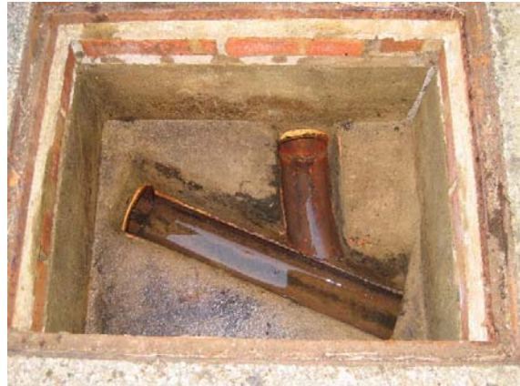
Typical inspection chamber
