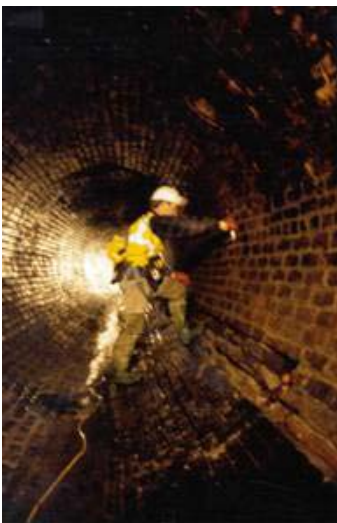
Figure 9 Inspecting for deterioration
