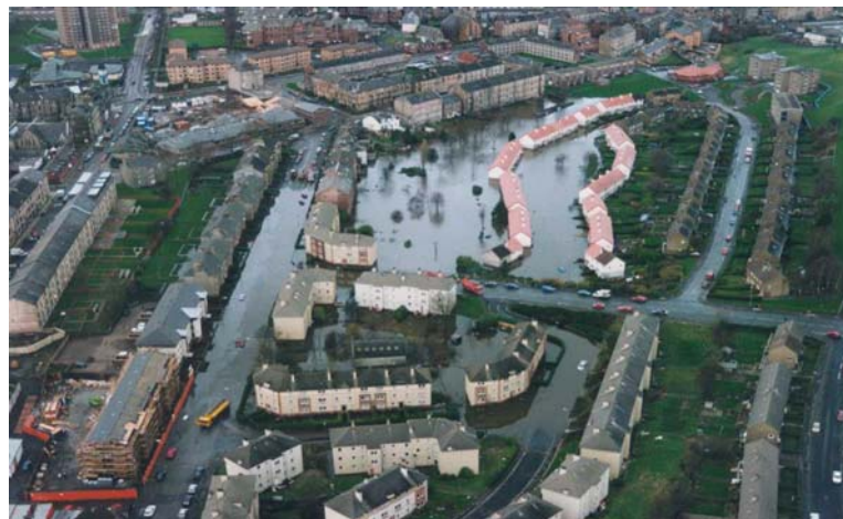
Figure 14 Flooding in Glasgow is not new - this is Paisley in 1994
