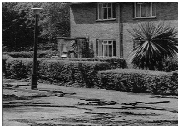
Figure 18 Effects of the Bracknell storm - properties flooded (above) and road surfaces scoured (below)
