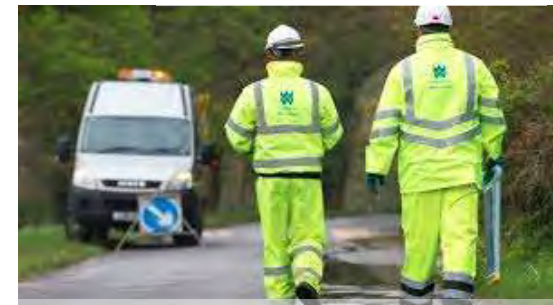
Sewer flooding investigations
