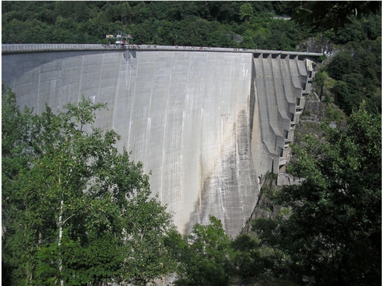
Verzasca Dam, Switzerland
