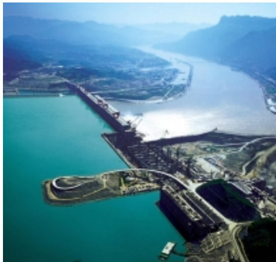
Three Gorges Dam, China
