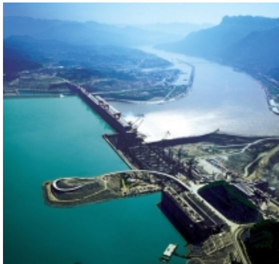
Three Gorges Dam, China
